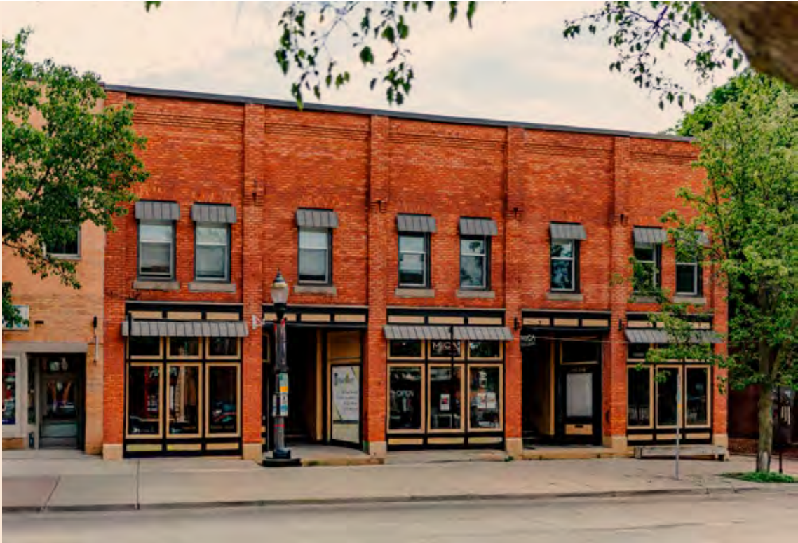
AFTER Turner Park building, 2026
